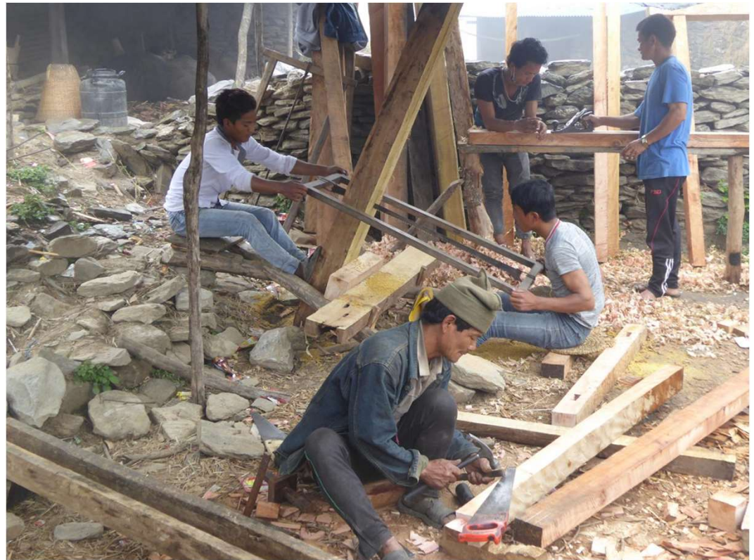
Housing reconstruction after the 2015 earthquake in Nepal © Bill Flinn, CARE UK
