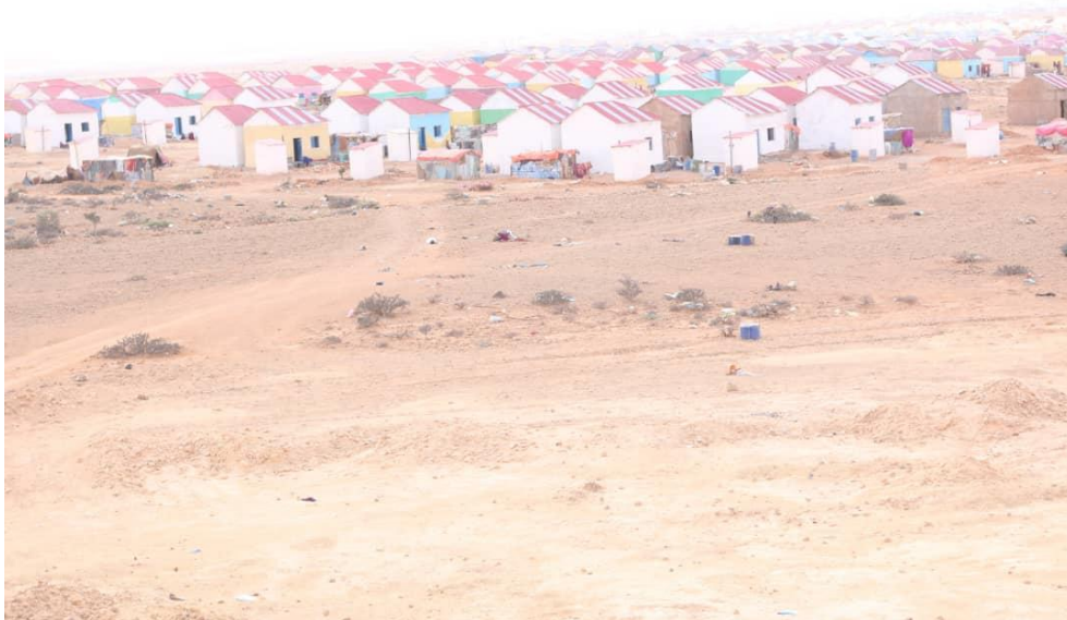
Permanent housing units for IDPs in Jilab 2 – NRC Garowe
