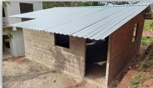
Roof and floor
