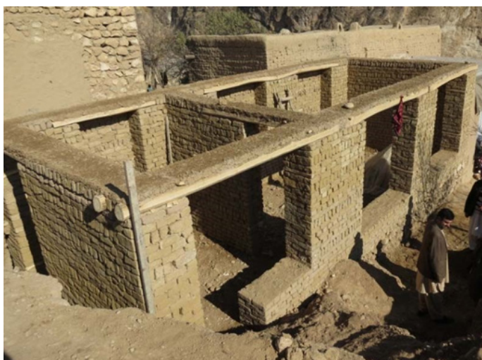
Preparation of roof plate
