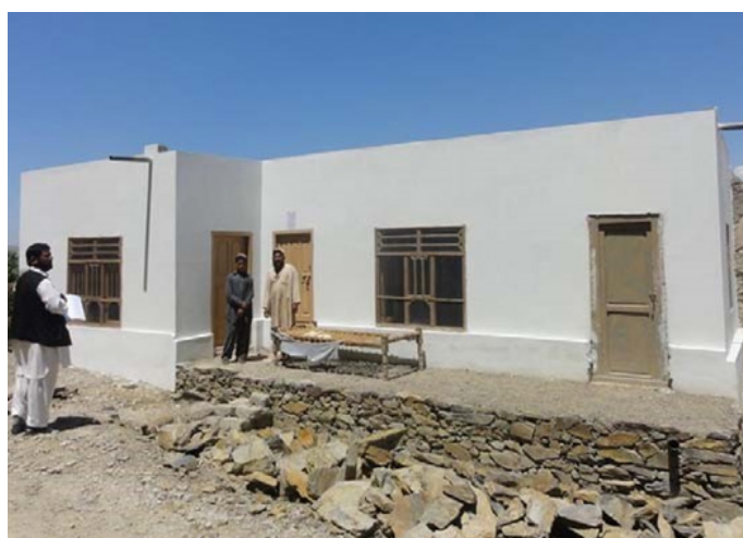
Shelter with doors and windows fitted, plastered
