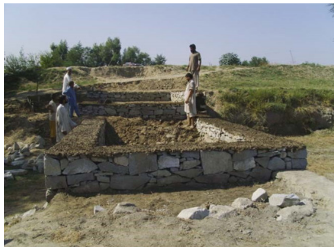
Cement mortar bound quarry rock foundation up to sill level (stone used in place of cooked brick).
