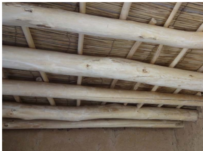
Installation of roofing materials
