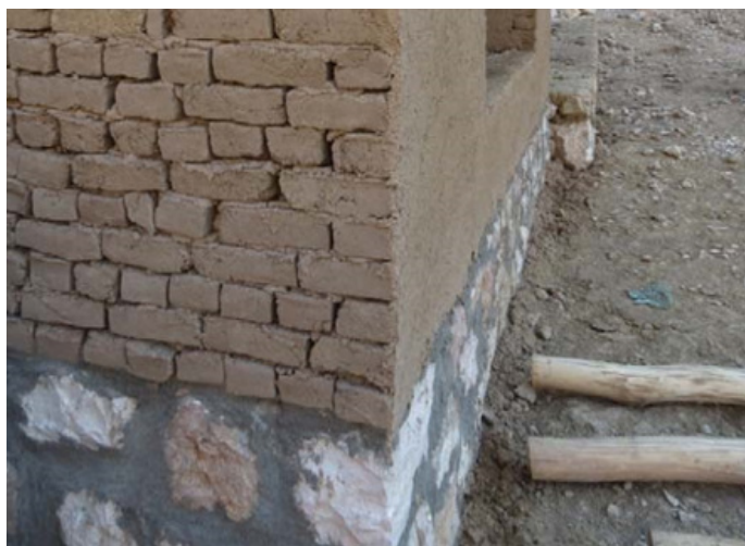
Cement mortar bound quarry rock foundation up to sill level (stone used in place of cooked brick).
