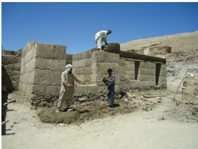
Pakhsa wall construction above lintel level
