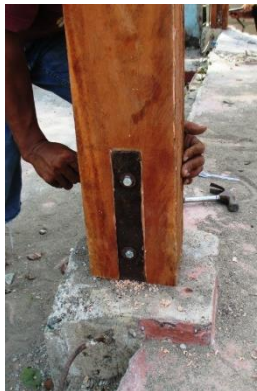
Left: The timber post is bolted to steel brackets cast into the concrete footing. Credit: CRS Owner-Driven Shelter construction, Barangay 58 Tacloban City (Photo: J. Girsang).
