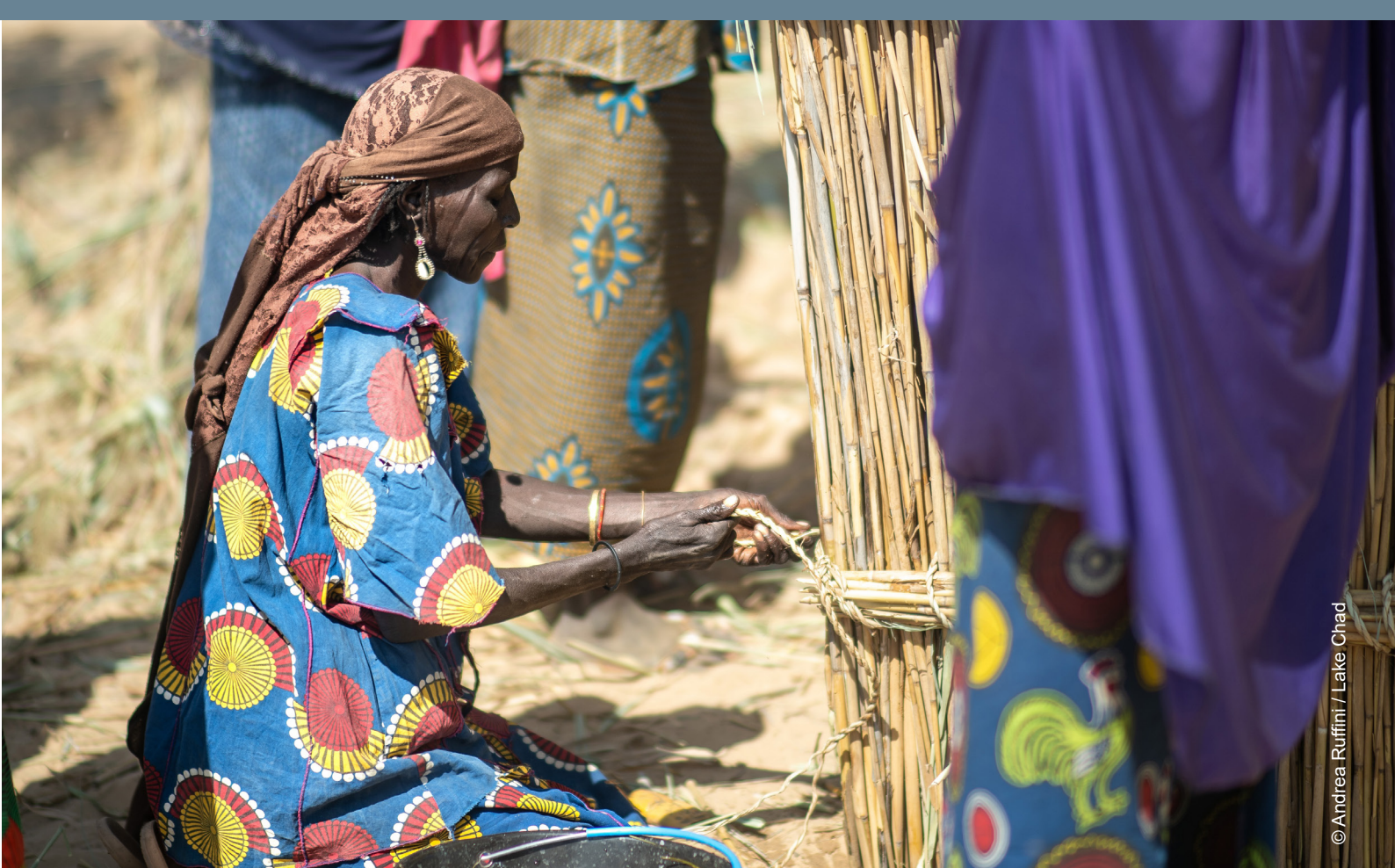
Woman interlacing straw during shelter construction.
