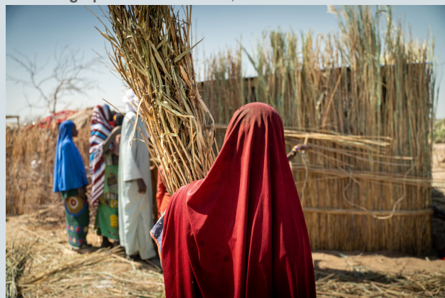
Women working on shelter construction providing straw.
