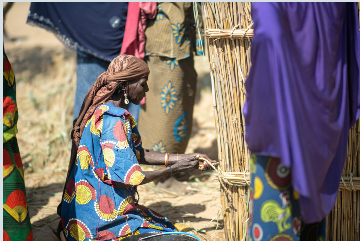
Woman interlacing straw during shelter construction.
