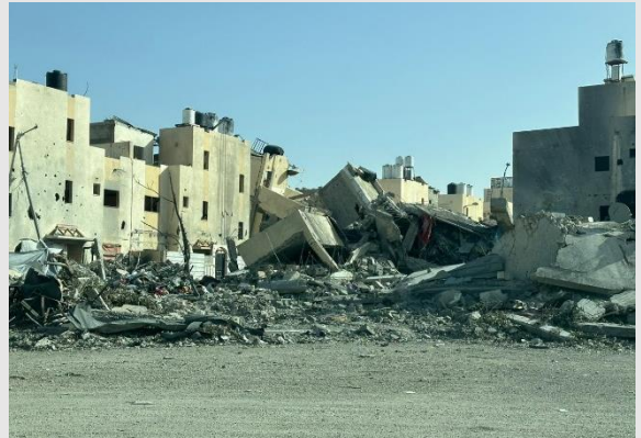
Destroyed building in Rafah, where the majority of IDPs have been displaced to. Photo: NRC/Mohammed Al Aklouk, Nov 2023.
