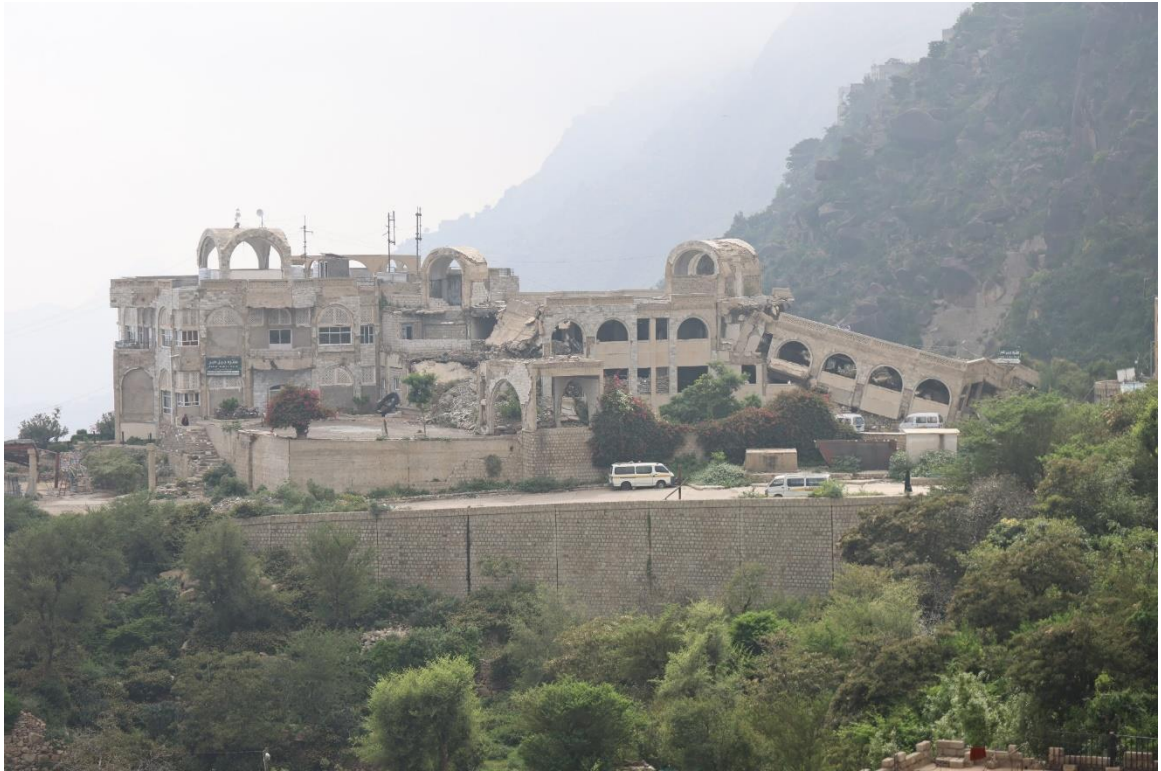
Fig 11-7 This once-popular public resting and viewing building in Saber Al Mawadim, Taiz, Now lies in ruins, heavily damaged by air strikes during the war, a stark reminder of the conflict's impact on the community.
