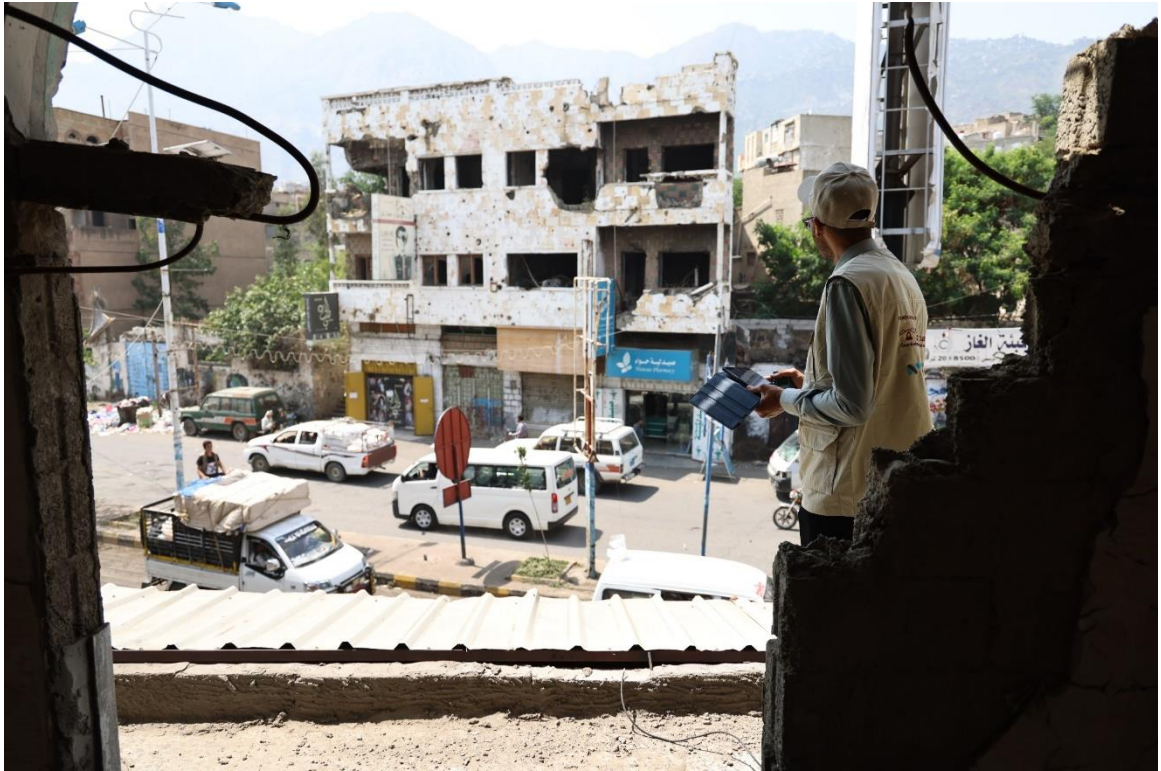
Fig 11-15 From a damaged building overlooking one of the most impacted main streets in Salah, Taiz, an NMO engineer evaluates the extent of destruction. Both sides of the street bear the scars of war, with buildings visibly damaged and in disrepair, underscoring the urgent need for rehabilitation and support in the community.
