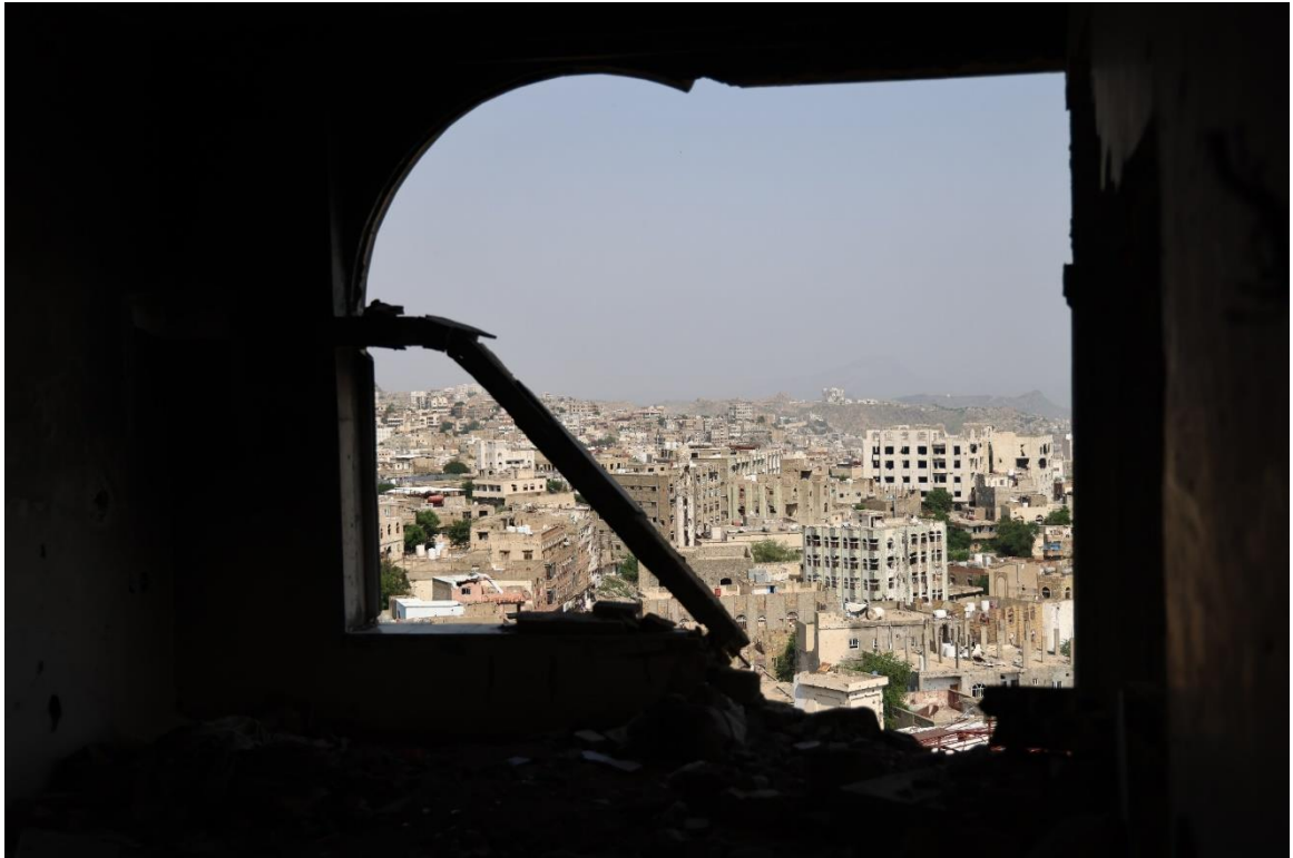
Fig 11-17 View from a damaged window in a building in Salah, Taiz, overlooking the war-torn landscape. The ruins of nearby structures reflect the impact of conflict on the community, showcasing the need for urgent rehabilitation efforts.
