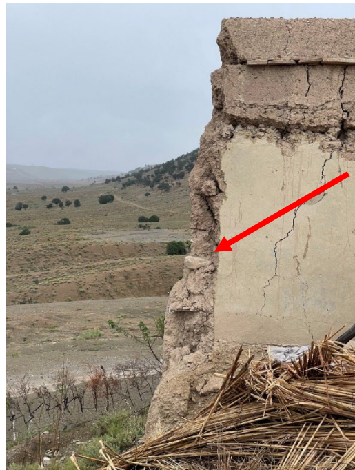
Figure 2-14. Failed section of Pakhsa wall
