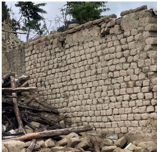
Figure 2-17 Example of poor mortar joints, poor rain protection and poor course work.
