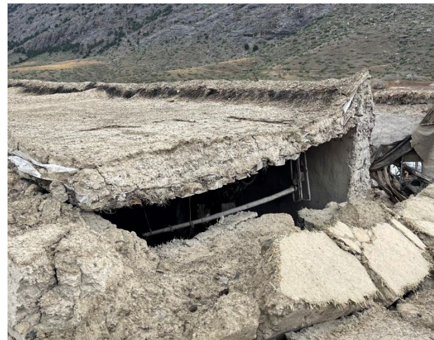
Figure 2-13. Failed section of multilayered roof.
