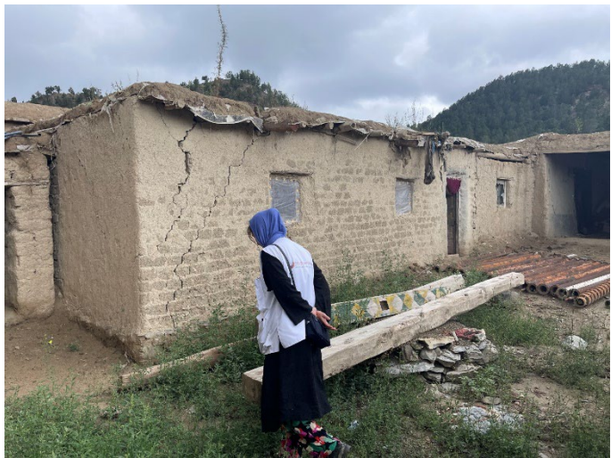
Figure 2-7 Example of mud brick construction.
