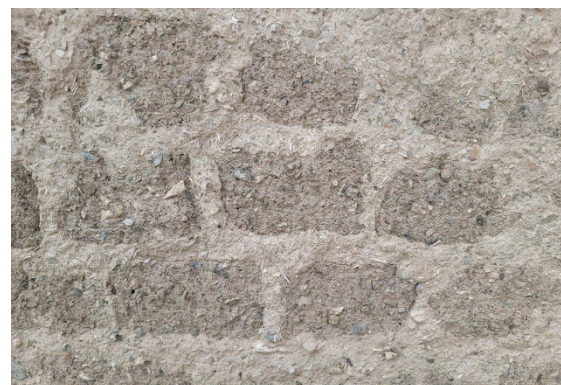
Figure 2-18. Example of plaster protecting mortar.
