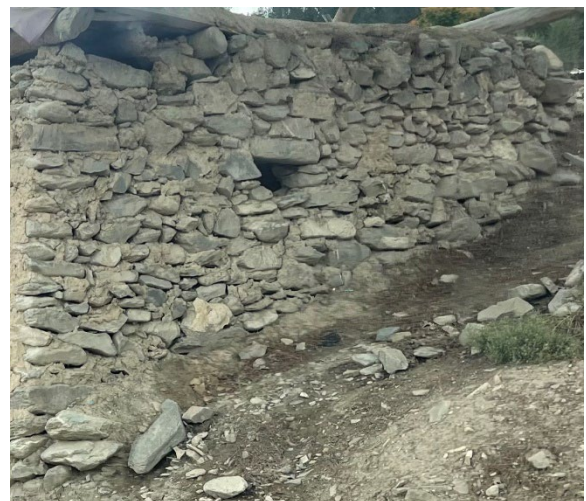
Figure 2-19. Example of angular rock wall construction.
