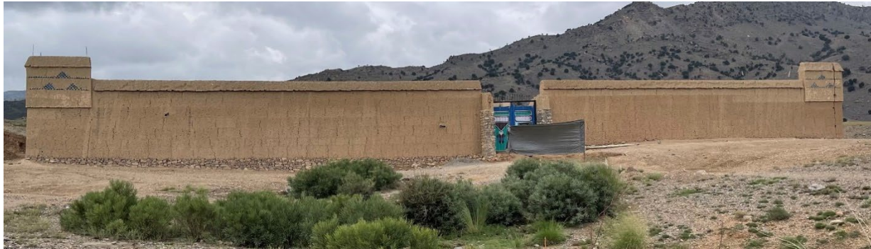
Figure 2-5. Example of a large Pakhsa compound wall (5-6m high).
