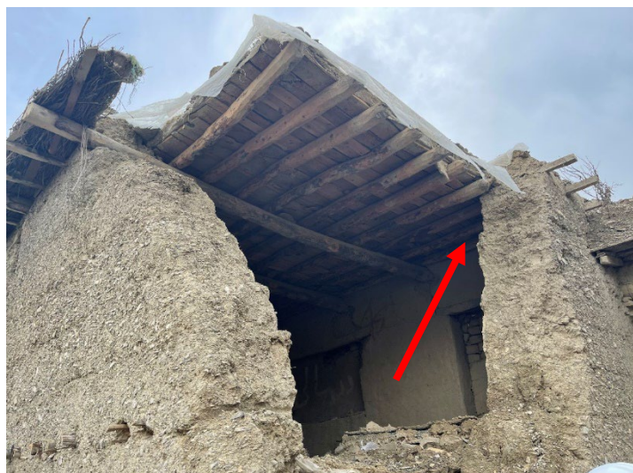
Figure 2-12 Example of Pakhsa wall construction
