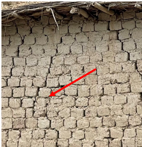
Figure 2-16. Example of insufficient coursing.
