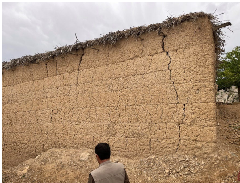
Figure 2-11 Example of commonly observed partial corner detachment.
