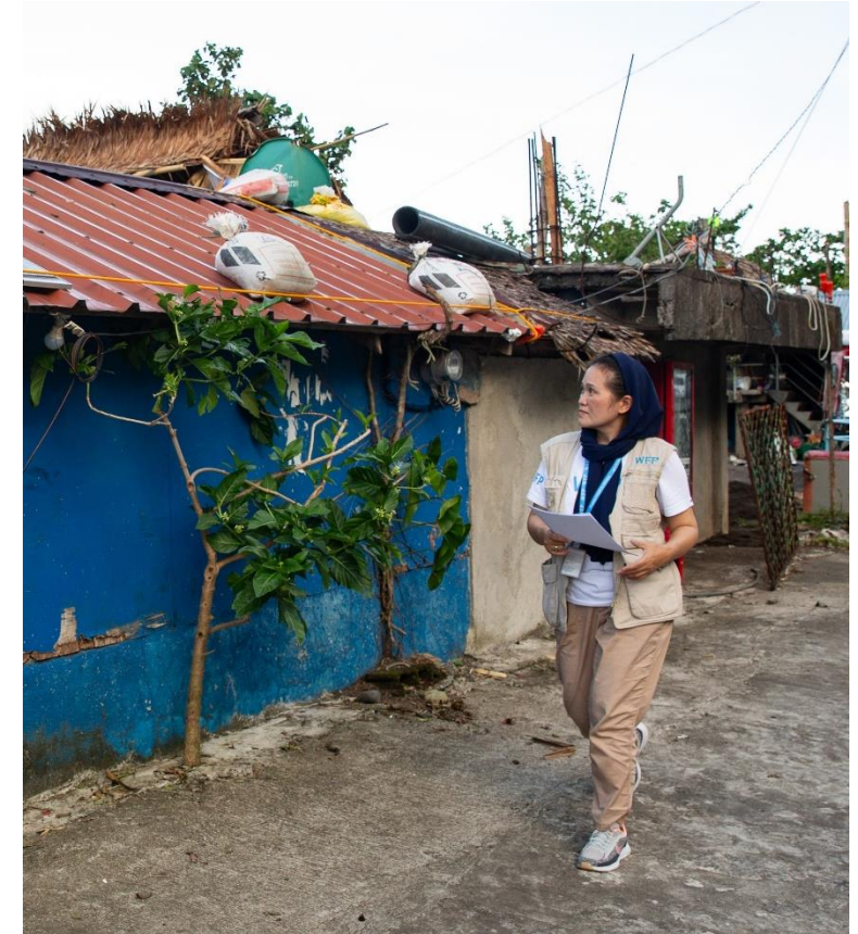
In Tiwi, Albay, WFP conducted a rapid damage assessment and needs analysis following the impacts of STY Pepito (Man-yi). © WFP/Earvin Perias
