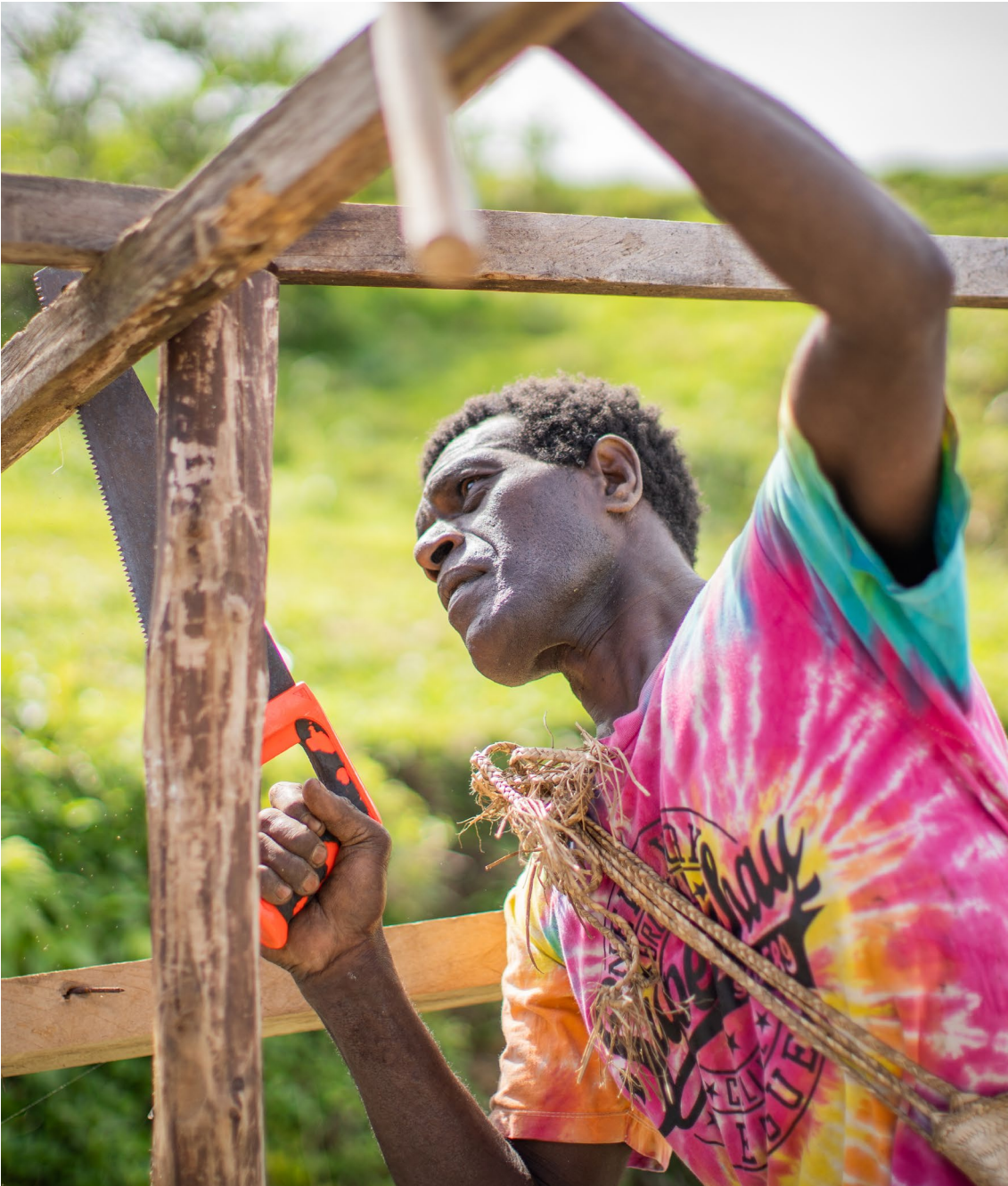
Rebuilding after Cyclone Harold, Vanuatu, 2020 Source: Valerie Fernandez
