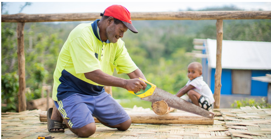
Rebuilding after Cyclone Harold, Vanuatu, 2020 Source: Valerie Fernandez
