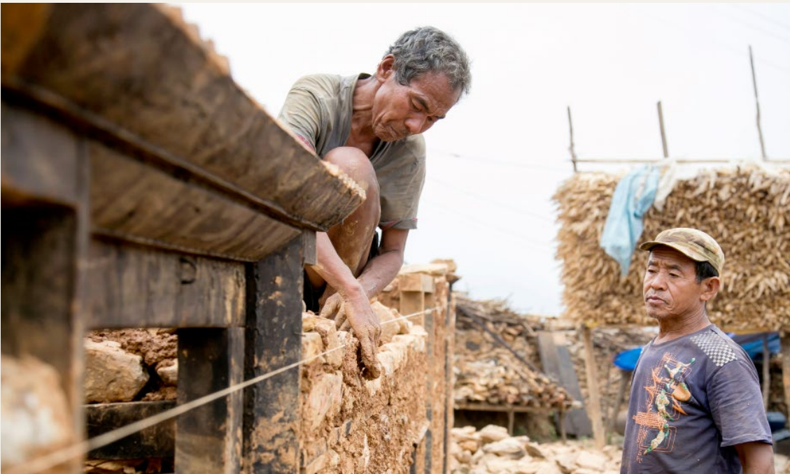
A local mason trained in earthquake resilient construction advises a householder as he reconstructs Source: Jennifer Hardy/CRS
