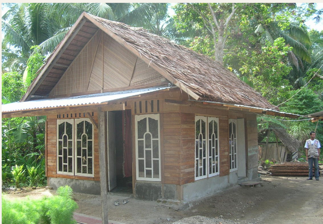
Transitional rebuilt house in Padang, Indonesia, using new and recycled material, 2009
