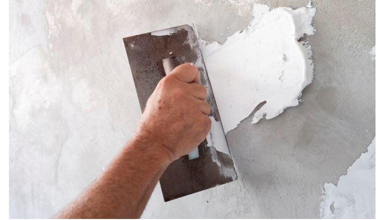
Crack Repairs
