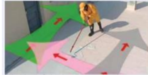
c. Applying the 2nd coat
