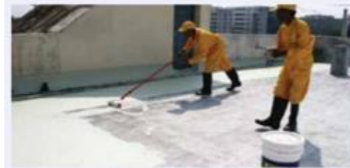
b. Applying the 1st coat
