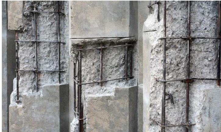
Crack Repairs
