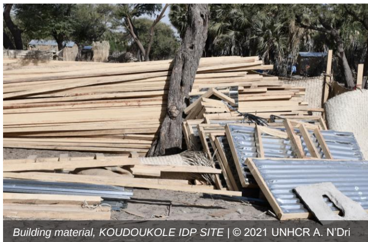
Semi-durable shelter construction, FOURKOLOM IDP SITE | © IOM
