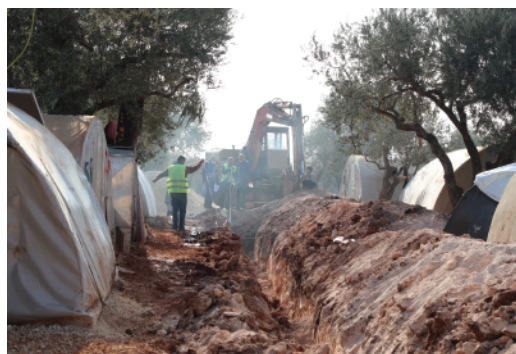
Infrastructure improvements in IDP sites. Photos: IYD
