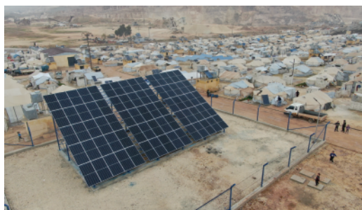
Infrastructure improvements in IDP sites. Photo: IOM
