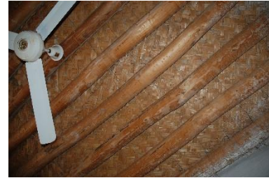
Ceiling sealing screen made with fibres mat — © CRAterre
