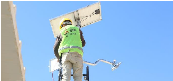
Solar panels installation, Arab Boran Camp – © Shafak
