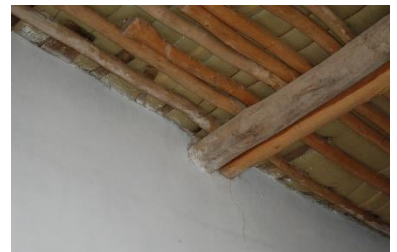
Wood structure (roof) – © CRAterre
