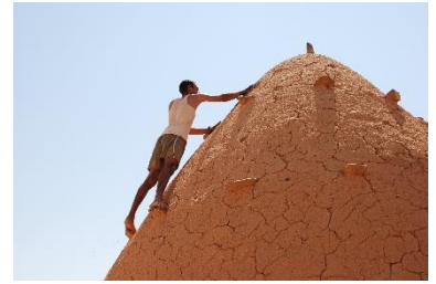
Maintenance: replastering – © CRAterre
