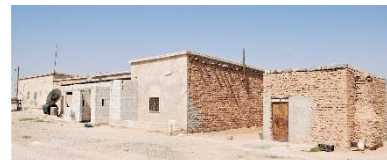
Concrete slabs and cement plasters over adobe load-bearing walls – © CRAterre
