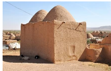
High dome with mud plaster – © CRAterre
