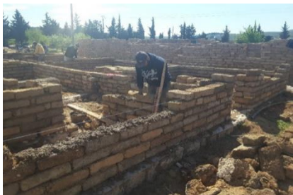
Al-Faroukia - construction site: adobe masonry (left); roofing (middle); plastering (right) – © QRC/BINAA
