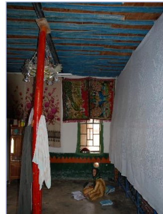
Intermediary metal I-beam to support joists for bigger width of room – © CRAterre
