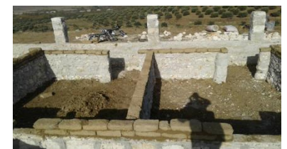
Btia – basement and start of adobe walls masonry – © QRC/BINAA
