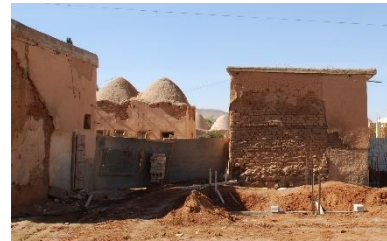
Concrete slabs over adobe load-bearing walls – © CRAterre
