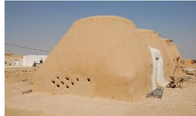
Holes left for ventilation – © CRAterre
