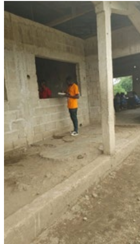
NRC School Repair
