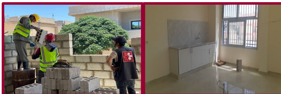
Left: Rehabilitation partially damaged apartment in Dar'a AL Balad, credit: PUI.
