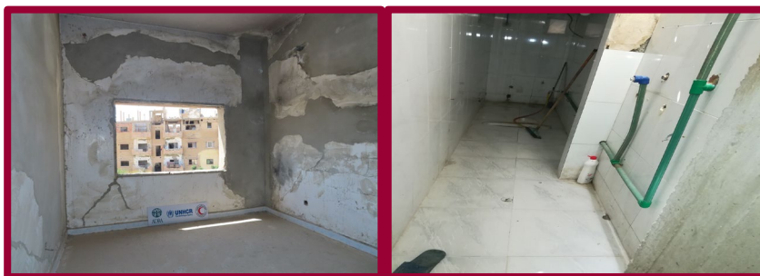
Left: Rehabilitation of damaged housing in Deir-ez-Zor city, credit: ADRA.
