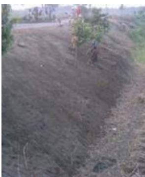
Slope for Vetiver plantation
