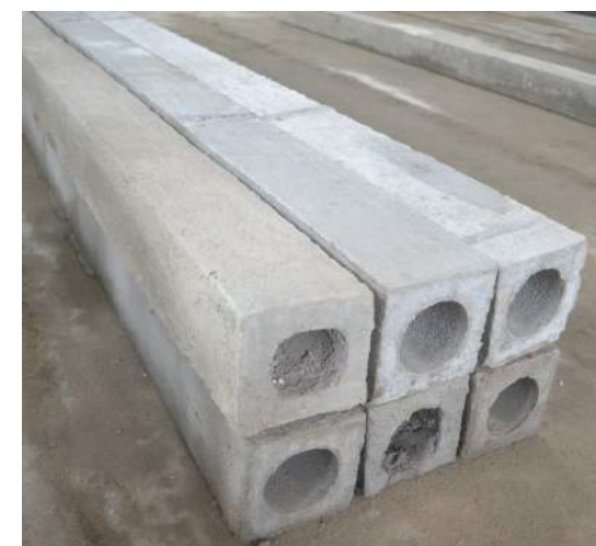
Ferrocement Hollow Column
