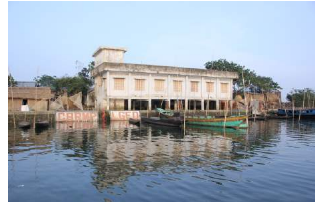
Protection with retaining wall
