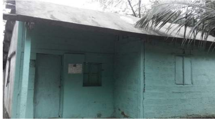
Cast in-situ Ferrocement Roof
