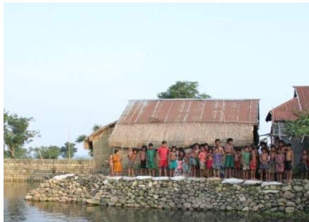
Protection with retaining walls and stones
