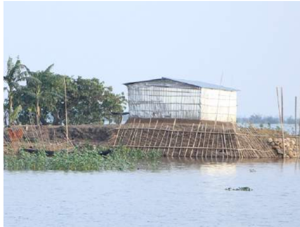
Protection with local stone and bamboo
