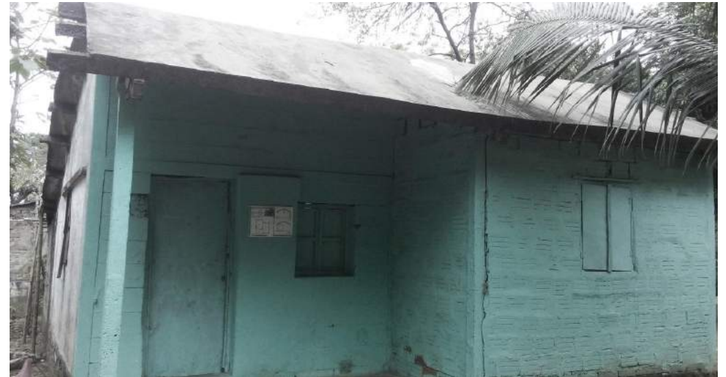
Cast in-situ Ferrocement Roof
