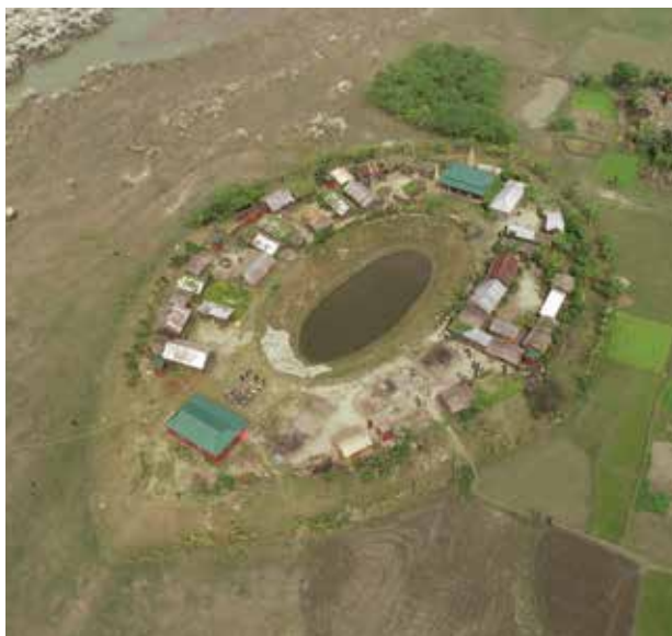
Picture: A cluster village on raised plinth; concept and constructed by Friendship Bangladesh.
