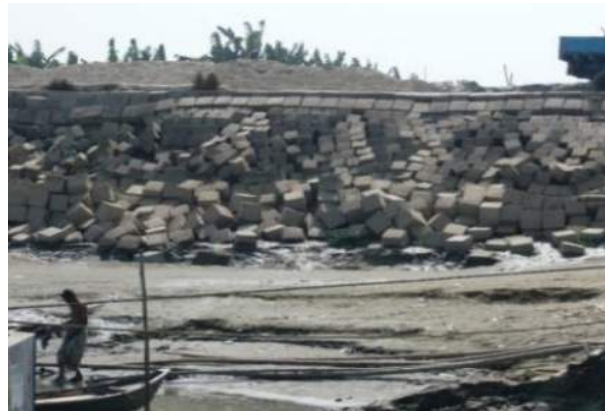
Concrete slope-stabilization blocks
