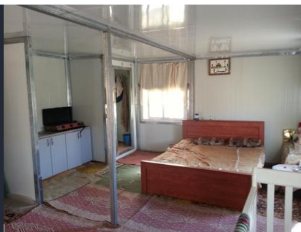
After the rehabilitation
