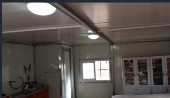
After the installation of solar energy system
