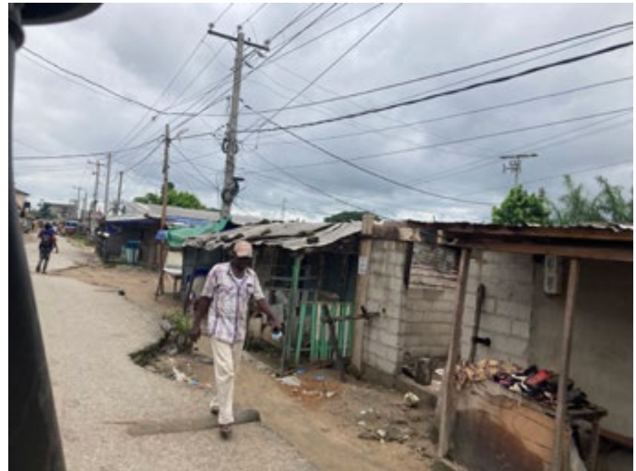
The village of Ndobbo in Douala 4, where many structures have been built along the road, despite building regulations stating that the building should be at least 5 m away from the road side. Buildings like these are often at risk of demolition.
