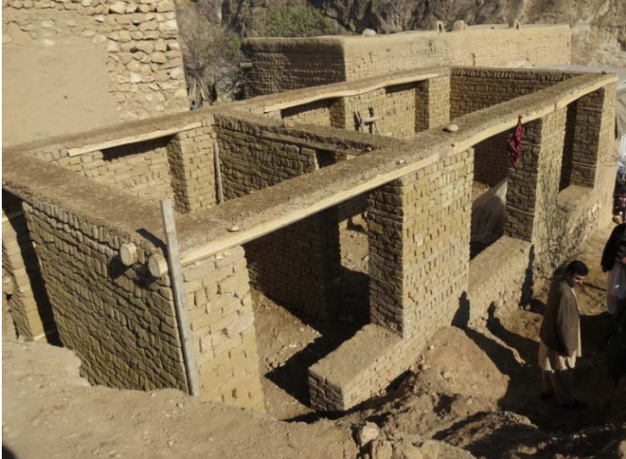
Preparation of roof plate.
