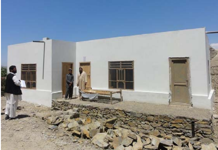
Shelter with doors and windows fitted, plastered and whitewashed.
