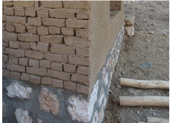
Cement mortar bound quarry rock foundation up to sill level (stone used in place of cooked brick).
