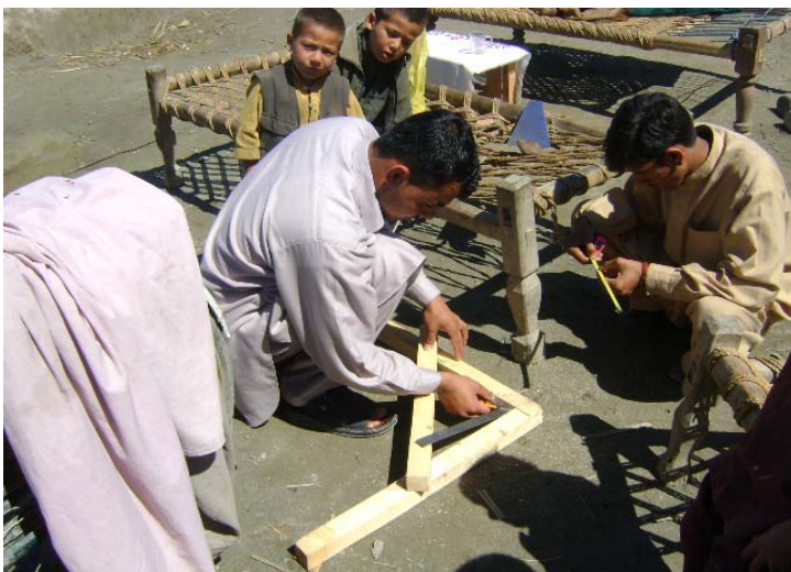
Fabrication of corner bracing for seismic mitigation.
