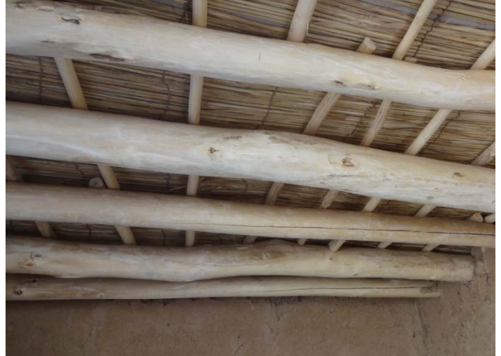
Installation of roofing materials.
