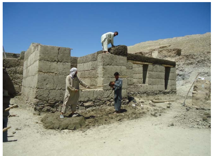
Pakhsa wall construction above lintel level.
