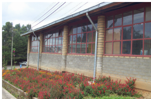
School built with CEB (Compressed Earth Blocks) in Addis Ababa. © O. Moles - CRAterre
