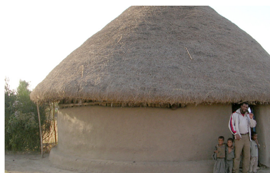
Ventilation is made possible thanks to the absence of plaster in the upper part of the walls in the Alaba houses (SNNPR). © Lorenzo Fontana
