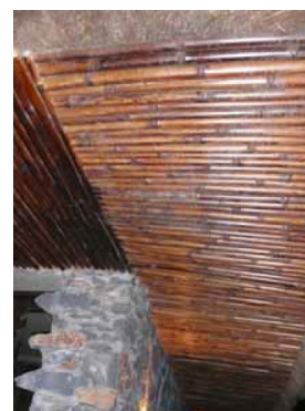
Bamboo ceiling near Bura (Amhara). Ceilings improve the house's comfort. © O. Moles- CRAterre
