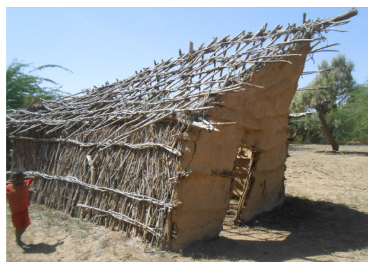
Rectangular house damaged by frontal undermining caused by standing flood water. © IOM- James Kennedy
