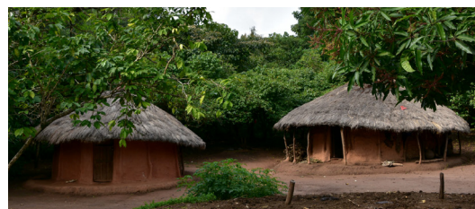
Aari houses built on a mound with a round verandah protecting the walls from the rain. (Debub Omo Zone in SNNPR). CC- Richard Mortel
