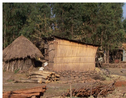
Constructions with stone plinths for protection of the wood and chikka walls from moisture and water splashing on the walls. (Amhara).
