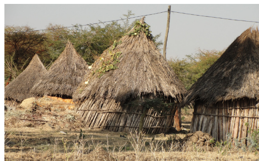
Stability problems due to black cotton soil expansion and contraction near lake Tana (Amhara). © L. Davis
