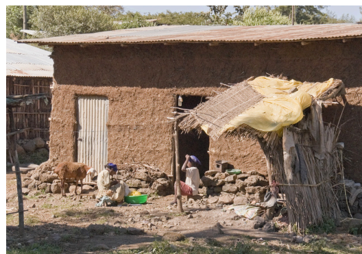
Stone masonry wall built to protect the lower part of the chikka walls in Bahir Dar. (Amhara). CC- A. Davey
