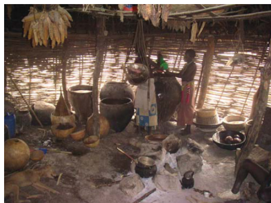
Interior ventilated space in a Gumuz house made of bamboo structure without chikka mortar and with a thatched roof. © A. González Ruibal et al.
