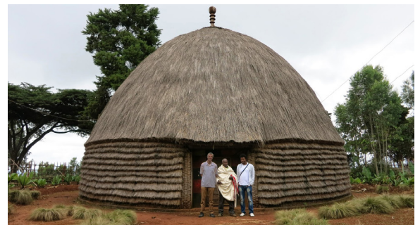
Welayta people house built with a bamboo structure and a vegetal covering. © Todd McGowan
