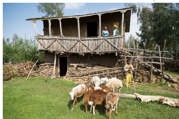
Two story house with stone plinth, chikka walls and balcony in Gobgob village, Amhara region. CC- Kelley Lynch USAID
