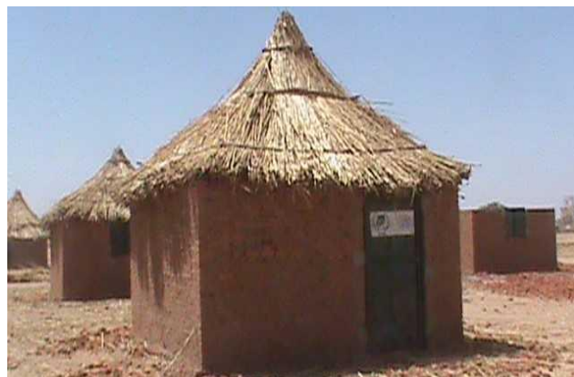
Transitional Shelter Project in Golo , Central Darfur
