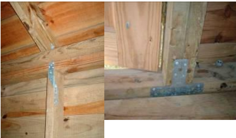
'T' strap used to connect the stud to the bottom plate.
