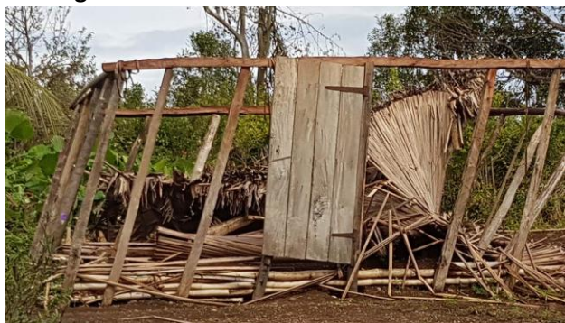
Shelter failure showing racking
