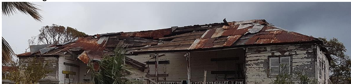
Failure of corrugated iron roofing
