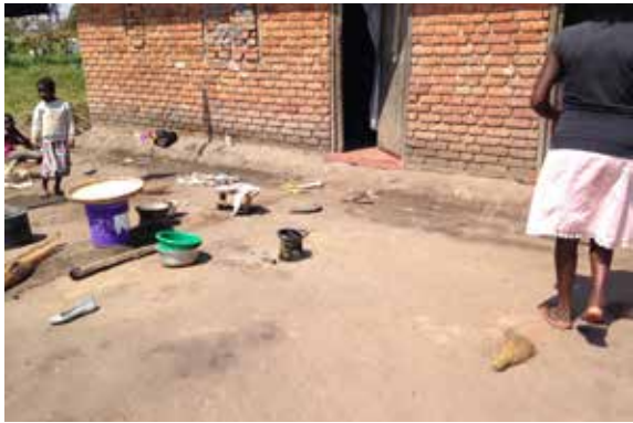
12. Small elevation of the floor level in floods prone areas.
