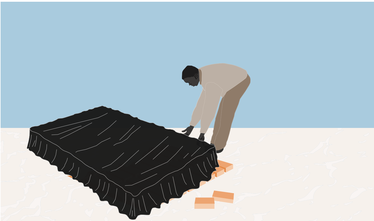
22. SSBs CURING UNDER PLASTIC SHEETS
