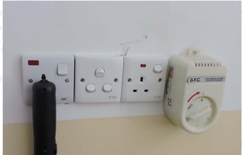
New electrical switches and plug points installed with electrical earth grounding.
