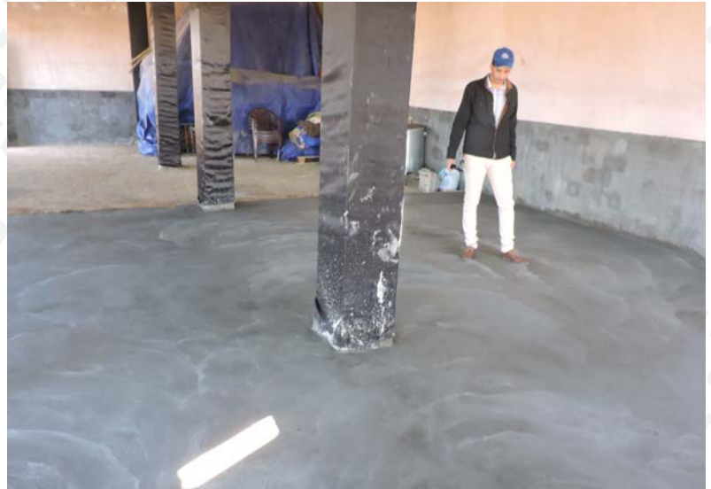
A family's living room floor is rehabilitated with 10cm reinforced concrete floor and structural column.
