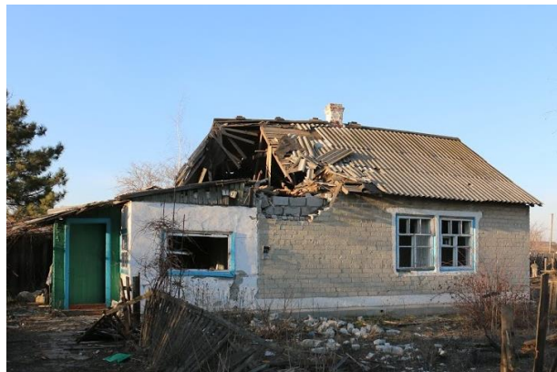
Figure 39 Brickwork with concrete block and burnt brick. People in Need assessment in Nikishine, 2015. credit R. Lunin
