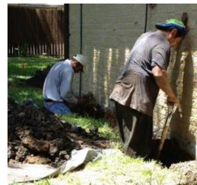
Figure 14 Digging pier hole checking
