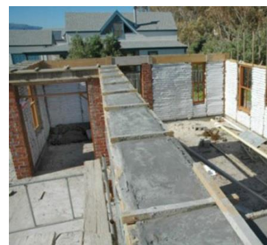
Figure 26. Concrete Casted upper ring beam, please note that concrete framework was not yet removed
