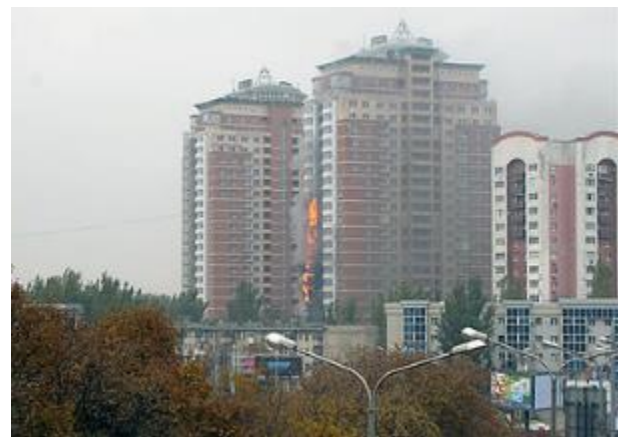
Figure 10 Fire in a multistoried building, donetsk 2015
