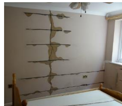
Figure 23 Wall stitches principle & pictures
