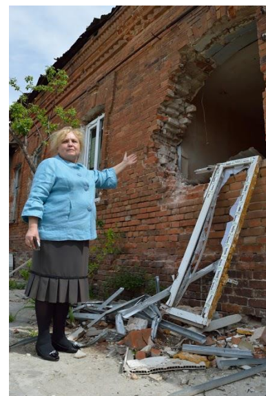
Figure 21 Replacement of windows, Sloviansk, People in Need 2015, credit R. Lunin
