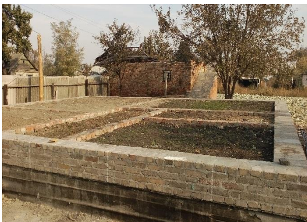
Figure 16 Reuse of the existing foundation for reconstruction. Please note that the foundation walls are excellent and don't need lower ring beam casting. Floor is not installed. (ADRA project Slovyansk 2015).
