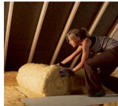
Figure 31 Insulation on attic floor, the volume of the attic increases the thermic performance
