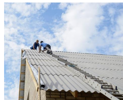
Figure 29 Asbestos free roofing material. People in Need, Sloviansk, 2016. Credit R Lunin
