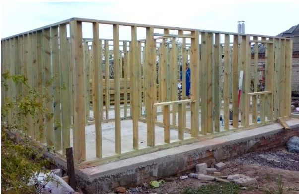
Figure 25 Timber framed wall inspired by North American Balloon Frame construction. Please note that wooden studs located on close interval are assembled as a panel as the load bearing structure. (Sloviansk, Dobraya Vest 2015)
