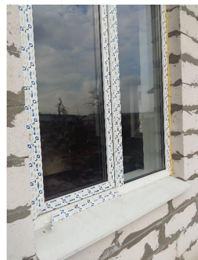
Figure 22 Windows, please note the insulation foam along the frame and the windows sill overhang in order to protect the wall. (Luxembourg Red Cross, Slovyansk 2015)
