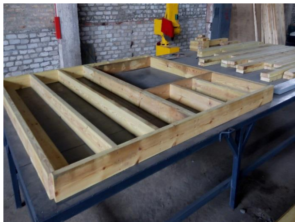
Figure 12 Pre fabrication of panels. Dobraya Vest 2016
