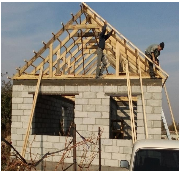
Figure 24 Concrete Block masonry, (Slovaisnk. ADRA 2015)
