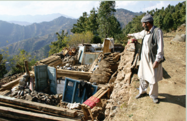
Narrow terraces, many houses include retaining walls.
