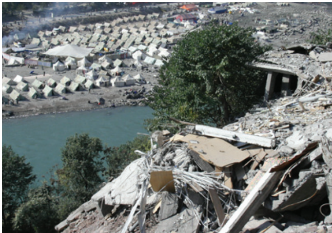
Muzaffarabad in 2005, extensive damage and displaced families.
