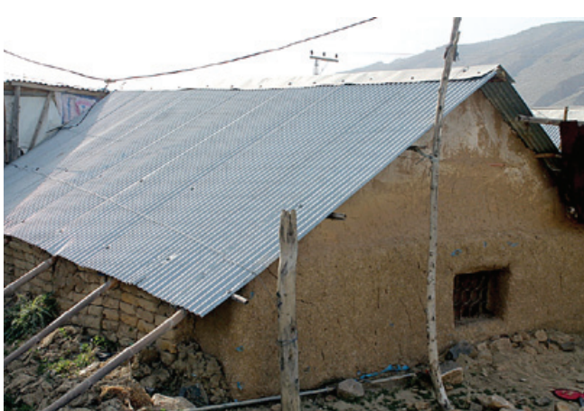
2015, T-shelter from 2008 with additional mud walling, no permanent reconstruction by this household.
