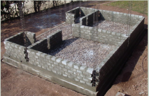
Confined masonry block construction, demonstration house.
