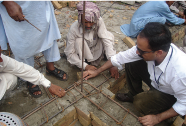
Ahsan explaining reinforcement details with masons.
