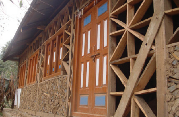
Masonry infilled timber frame, local techniques regenerated.
