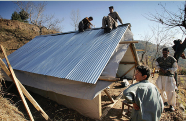
Constructing demonstration shelter, 2005.
