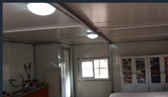
After the installation of solar energy system
