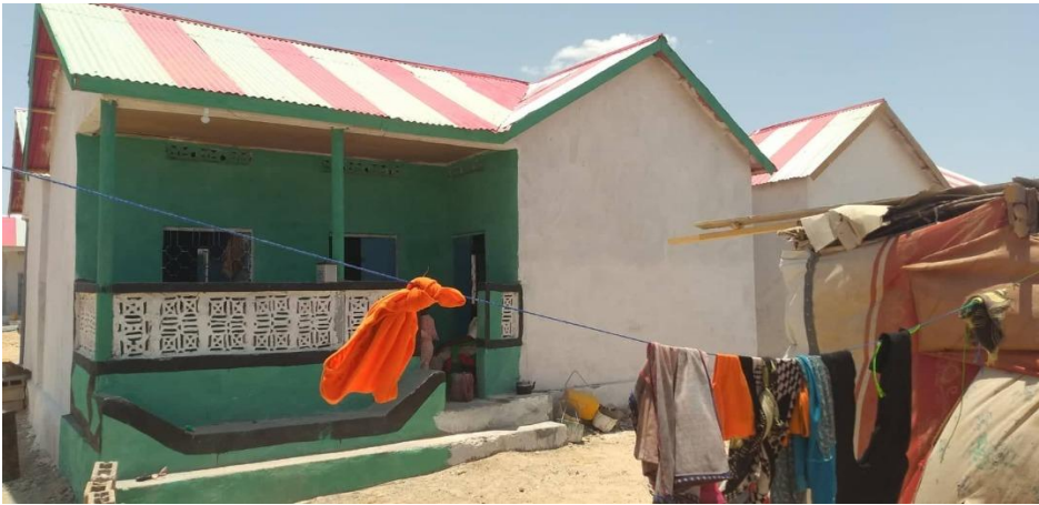
Stone/brick wall with CGI roof: Type 1 Derbiga Stone / bulukeeti saqafka CGI: Nooca 1
