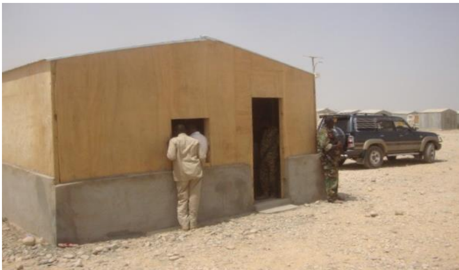
Plywood wall with CGI roof / Darbiga plywood oo leh saqafka CGI
