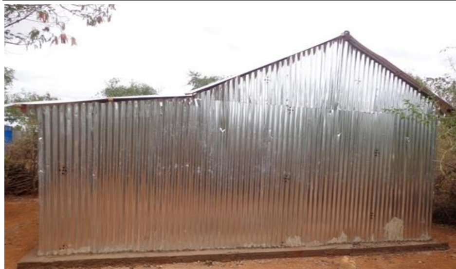
CGI sheet wall and roof / CGI sheet iyo saqafka.
